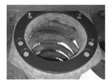
Mark the four holes on the outer edge of the ring. Drill these through with a 9mm drill.
